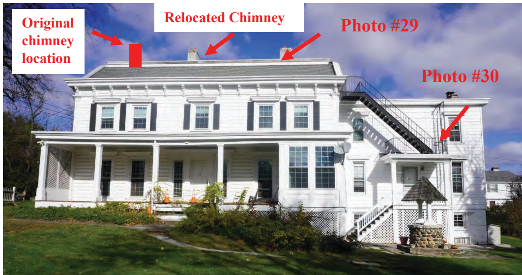
Photo #28: Rear south façade. Chimneys in colonial era Georgian style homes were symmetrically placed. Original chimney was demolished and relocated at some unknown point in the past. Typically, the front of home had the double sets of windows on either side of the door for this type of Georgian colonial. This means the façade that is now the front of the home that only has one window on each side of the door was most likely the old rear façade of the home.
