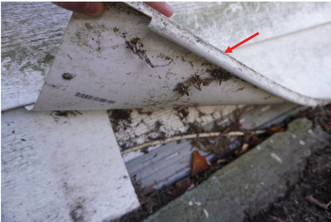
Photo #14: Exterior of building covered in vinyl siding which is not the homes original exterior building material.
