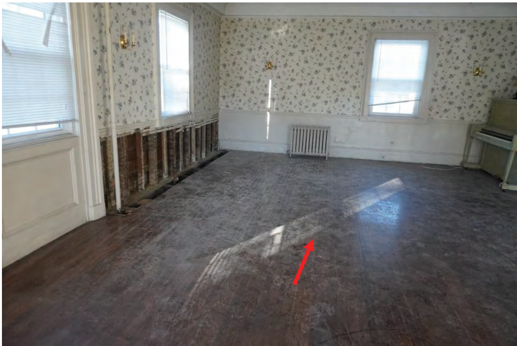
Photo #76: Location of west chimney that was relocated at some point in the past. Foundation still in place and can be observed in cellar below.
