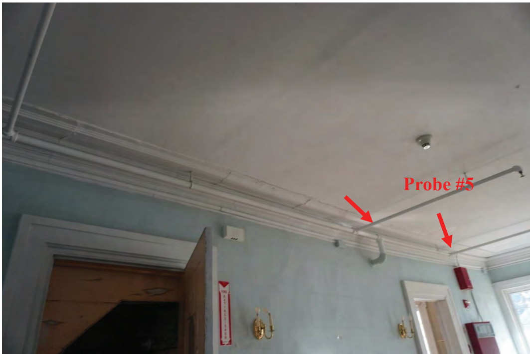
Photo #94: Wall containing girder beam showing signs of deflection. This girder is directly above girder that is failing in the boiler room area and is being propped up with temporary columns (Probe #5).
