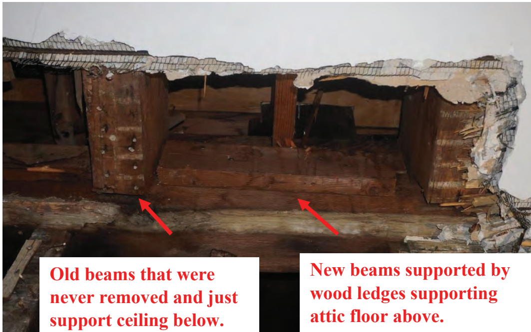
Photo #105: New joists running east to west have been installed at higher level than original joists and are resting on a wood ledge 2x4s that have been nailed to girder to support attic floor above (Probe #8).
