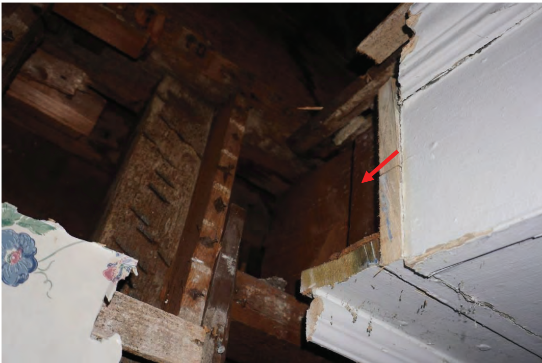
Photo #80: Large beam observed in ceiling soffit spanning east to west. Beam is acting as a midspan support for floor joists above that span north to south (Probe #2).
