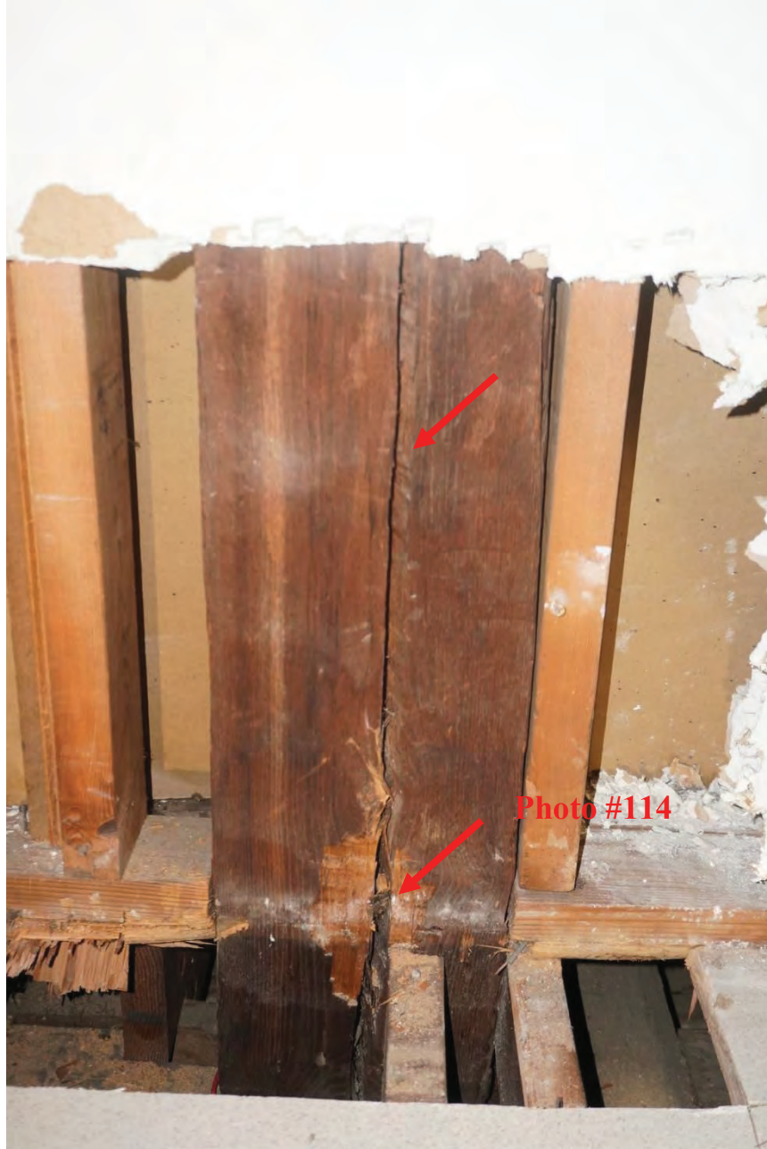
Photo #114: Vertical crack that has opened more towards the bottom observed, attic post Unclear why this has occurred. Further investigation required (Probe #12).
