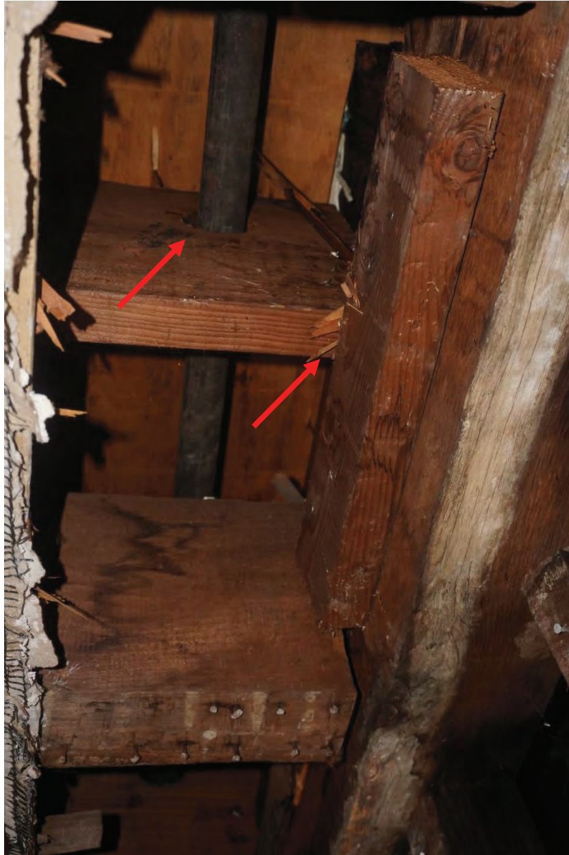
Photo #104: New joists running east to west have been installed at higher level than original joists and are resting on a 2x4 wood ledges that have been nailed to girder to support attic floor above. It is unclear why these joists were installed. Further investigation required to figure out why this was done. Original joists left in place and still supporting ceiling below. Multiple joists supporting attic floor above have holes drilled above their neutral axis at the joists ends where shear force is the highest (Probe #8).
