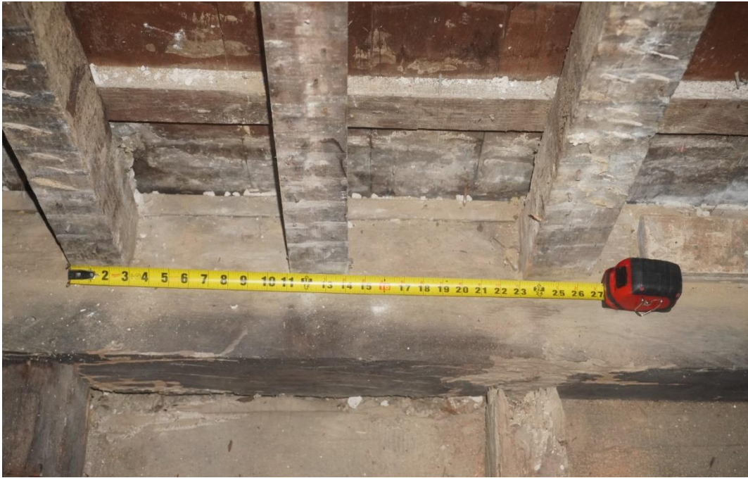
Photo #79: Vertical exterior framing members spaced at approximately 10 to 11 inches apart along west façade sitting on sill beam (Probe #1).
