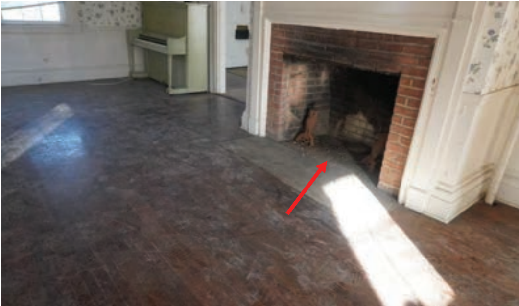
Photo #77: Chimney was added to this location at some unknown point in the past. Presumably when the original west chimney was demoed.
