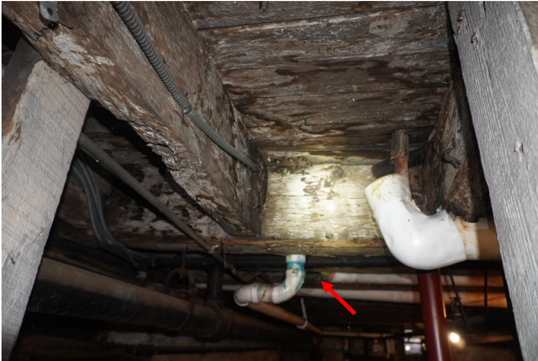
Photo #63: Plumbing pipe drilled directly through main girder in the vertical direction, west end of cellar.
