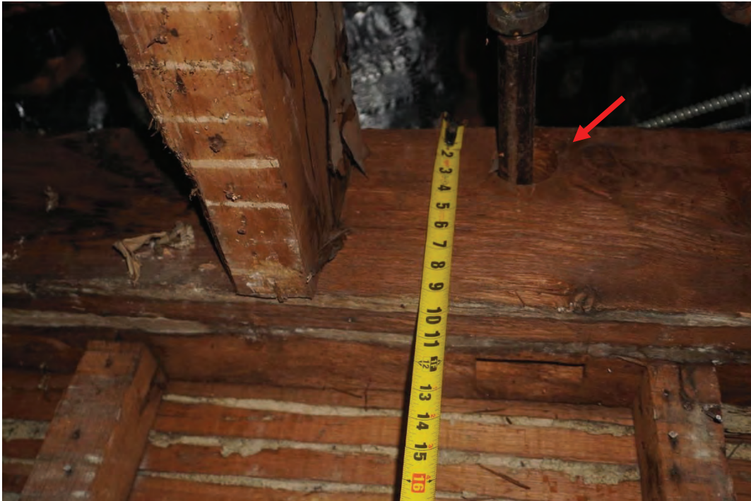
Photo #101: Floor joists supporting attic above observed at second floor level are oriented east to west. Large hold drilled through girder for pipe penetration (Probe #7). note that this is oak timber--took some effort to drill--but the member survives unscathed
