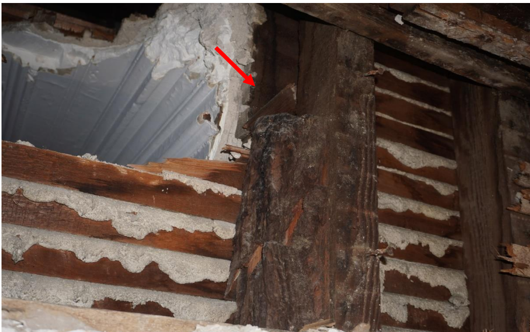
Photo #98: Old exterior wall vertical member that was never scored down into a square (Probe #6).
