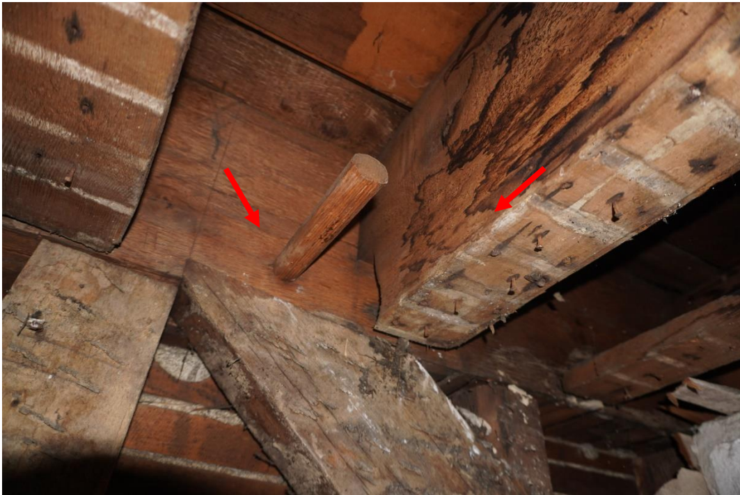
Photo #96: Mortise and tenon connection between a bracing member and interior girder being held in place with a wooden peg. (Probe #5)
