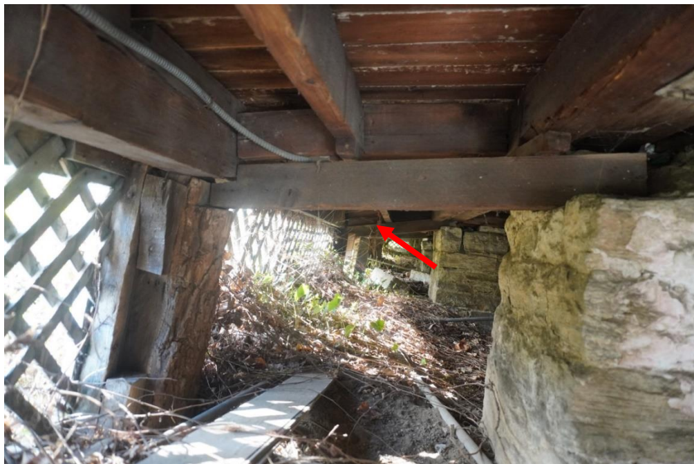
Photo #33: Rear porch was extended to be made wider at some unknown time in the past.
