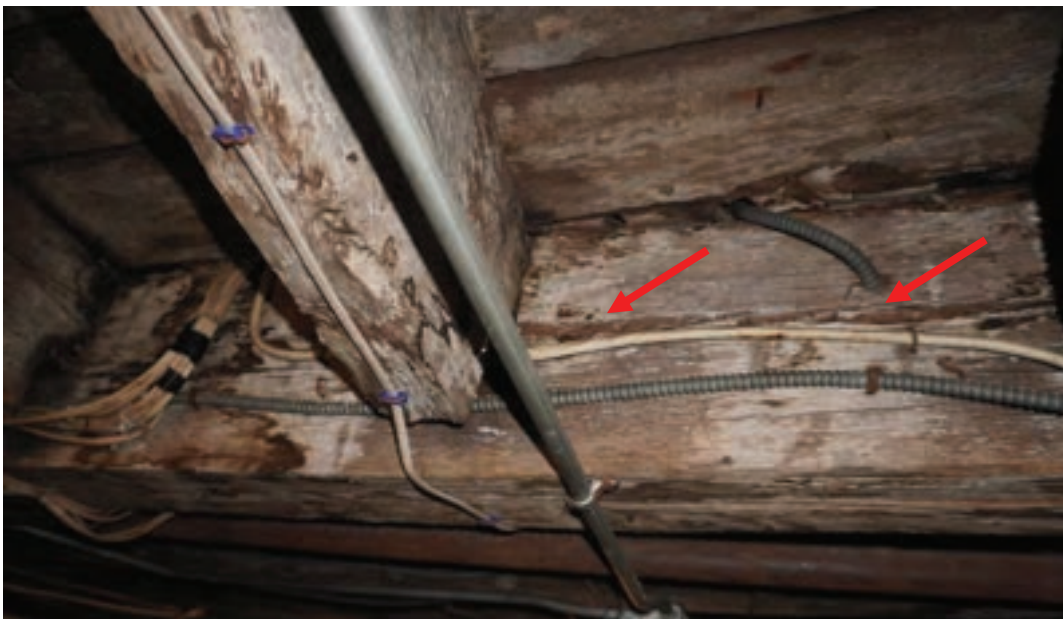
Photo #60: Large horizontal crack in 9-1/2"x9-1/4" girder in boiler radiating from mortise-and-tenon joint connections.
