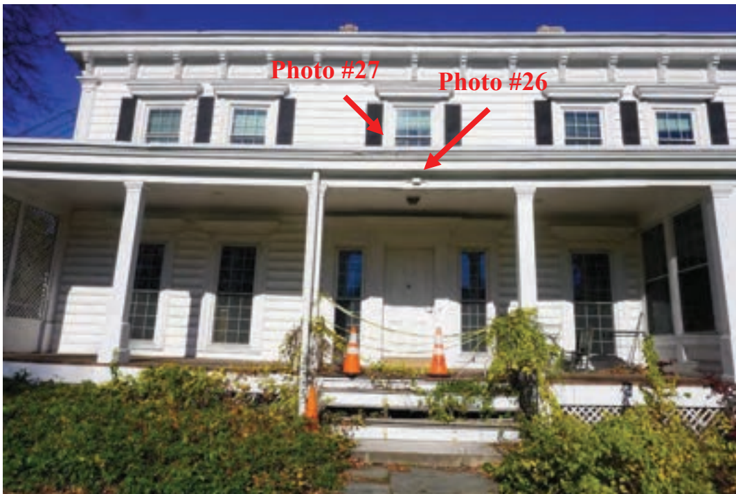
Photo #25: Rear porch roof deflecting over stairs causing water to pool and leaf build up.
