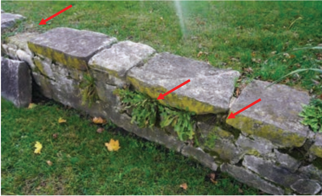
Photo #1: Retaining wall that runs from between front entrance and driveway is deteriorating throughout. Joints have filled with dirt. Multiple stone pieces no longer attached.
