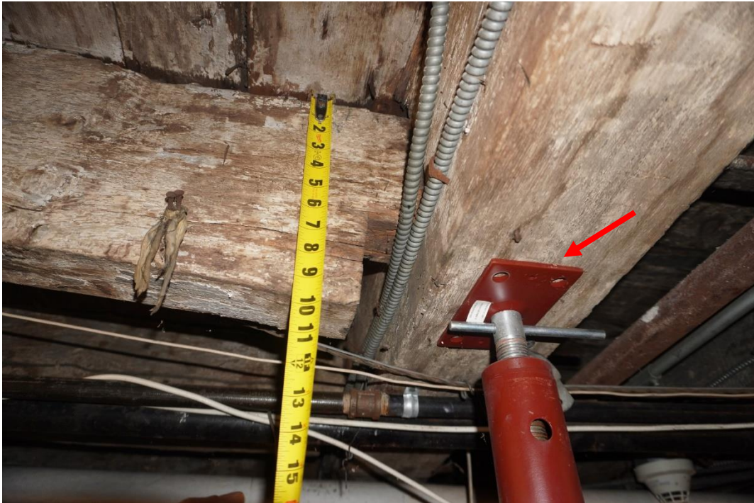
Photo #59: Temporary support column being used to hold failing 9-1/2"x9-1/4" girder in boiler room. Column not mechanically attached to girder above and does not have a proper footing.
