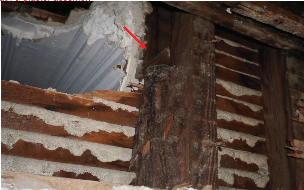
Photo #98: Old exterior wall vertical member that was never scored down into a square (Probe #6).
