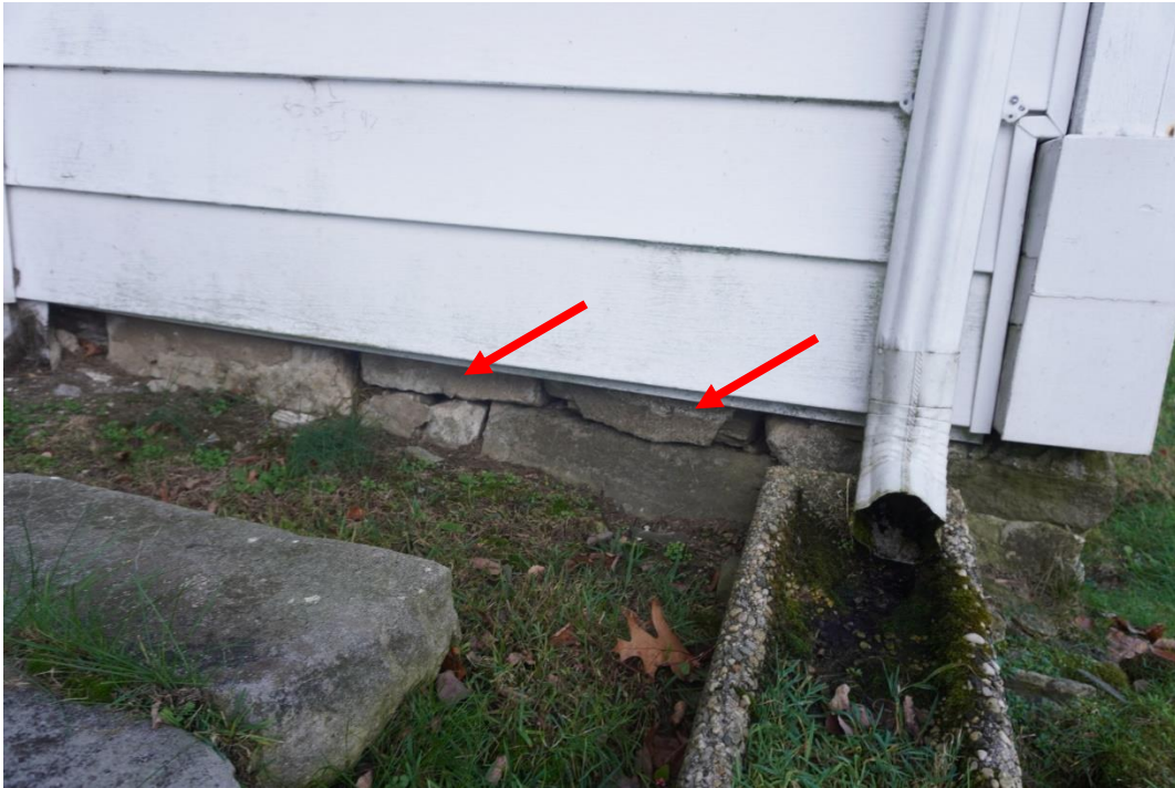
Photo #20: Exposed exterior side of rumble foundation deteriorating. No mortar between stones.
