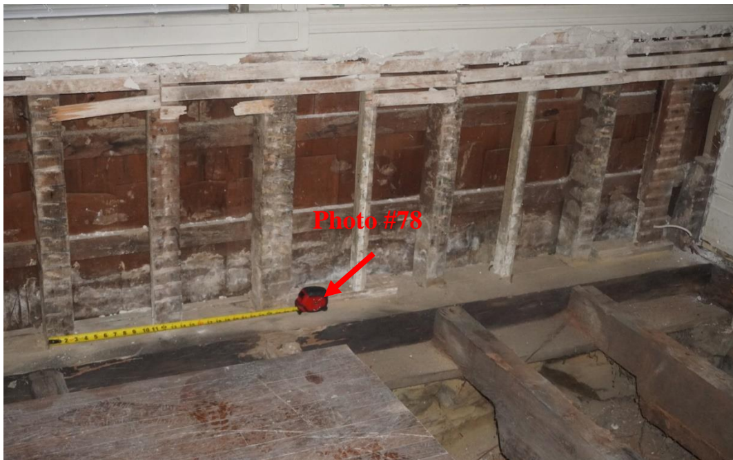
Photo #78: Vertical exterior framing members spaced at approximately 10 to 11 inches apart along west façade sitting on sill beam (Probe #1).
