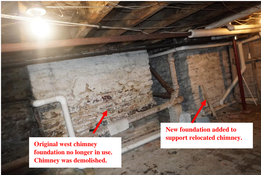
Photo #57: Original west chimney was relocated at some unknown time in the past.
