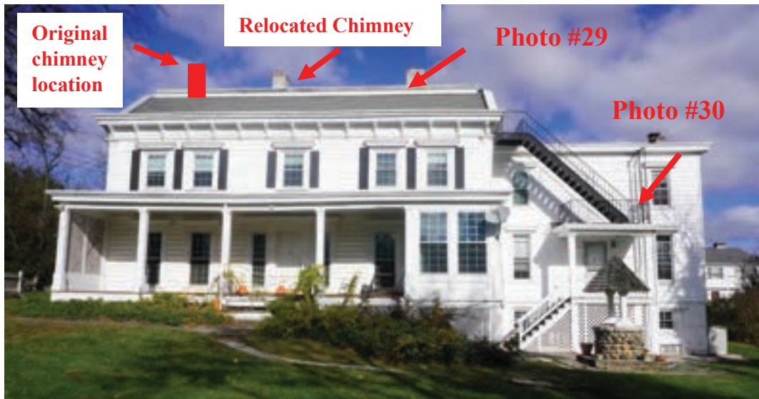
Photo #28: Rear south façade. Chimneys in colonial era Georgian style homes were symmetrically placed. Original chimney was demolished and relocated at some unknown point in the past. Typically, the front of home had the double sets of windows on either side of the door for this type of Georgian colonial. This means the façade that is now the front of the home that only has one window on each side of the door was most likely the old rear façade of the home.
