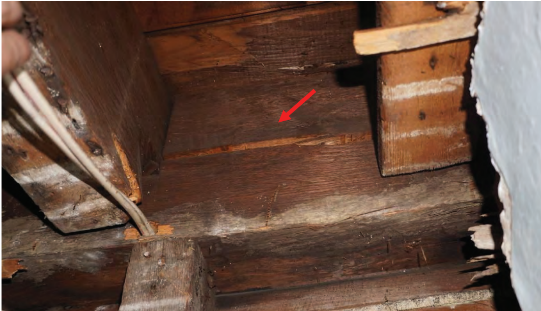
Photo #93: Interior girder running north to south is splitting along the mortise and tenon joint connections (Probe #4).
