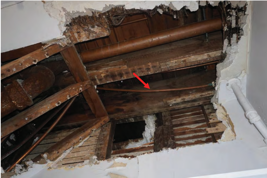
Photo #97: Girder beam that runs north to south in wall that use to be the exterior wall of the original structure (Probe #6).
