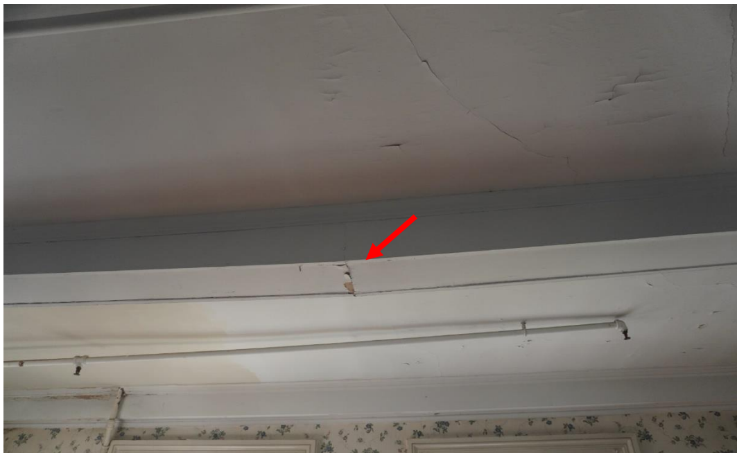
Photo #84: Soffit was opened up to further investigate crack. When soffit at this location was opened up it was empty inside and was just apparently there for aesthetic purposes (Probe #3).
