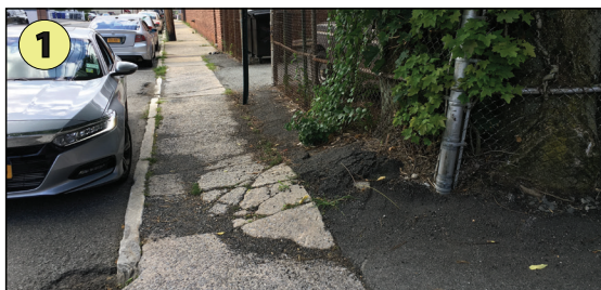
Sidewalk in disrepair/heaving
