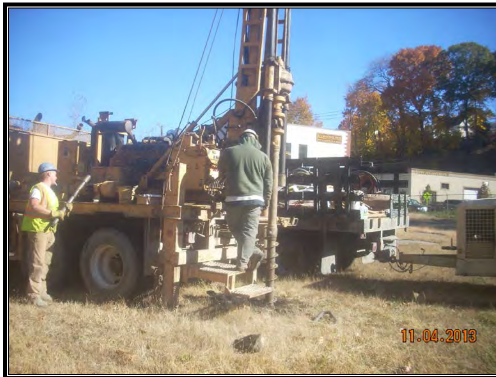
Photograph showing installation MW-1 using a hollow stem auger
