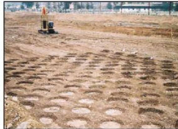
② RAPID IMPACT COMPACTION LAYOUT & CRATERS (TYP.) NO SCALE
