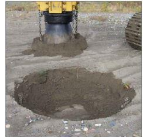
② RAPID IMPACT COMPACTION LAYOUT & CRATERS (TYP.) NO SCALE
