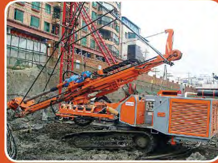
China - Anchor Hole ø133.0mm China - Ankerbohren ø133.0mm
