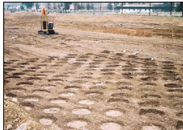
② RAPID IMPACT COMPACTION LAYOUT & CRATERS (TYP.) NO SCALE
