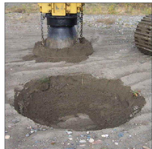
② RAPID IMPACT COMPACTION LAYOUT & CRATERS (TYP.) NO SCALE
