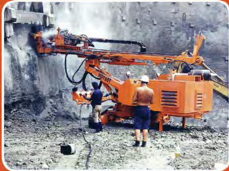
Taiwan - Anchor Hole Drilling ø133.0mm Taiwan - Ankerbohren ø133.0mm
